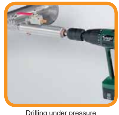
Drilling under pressure
